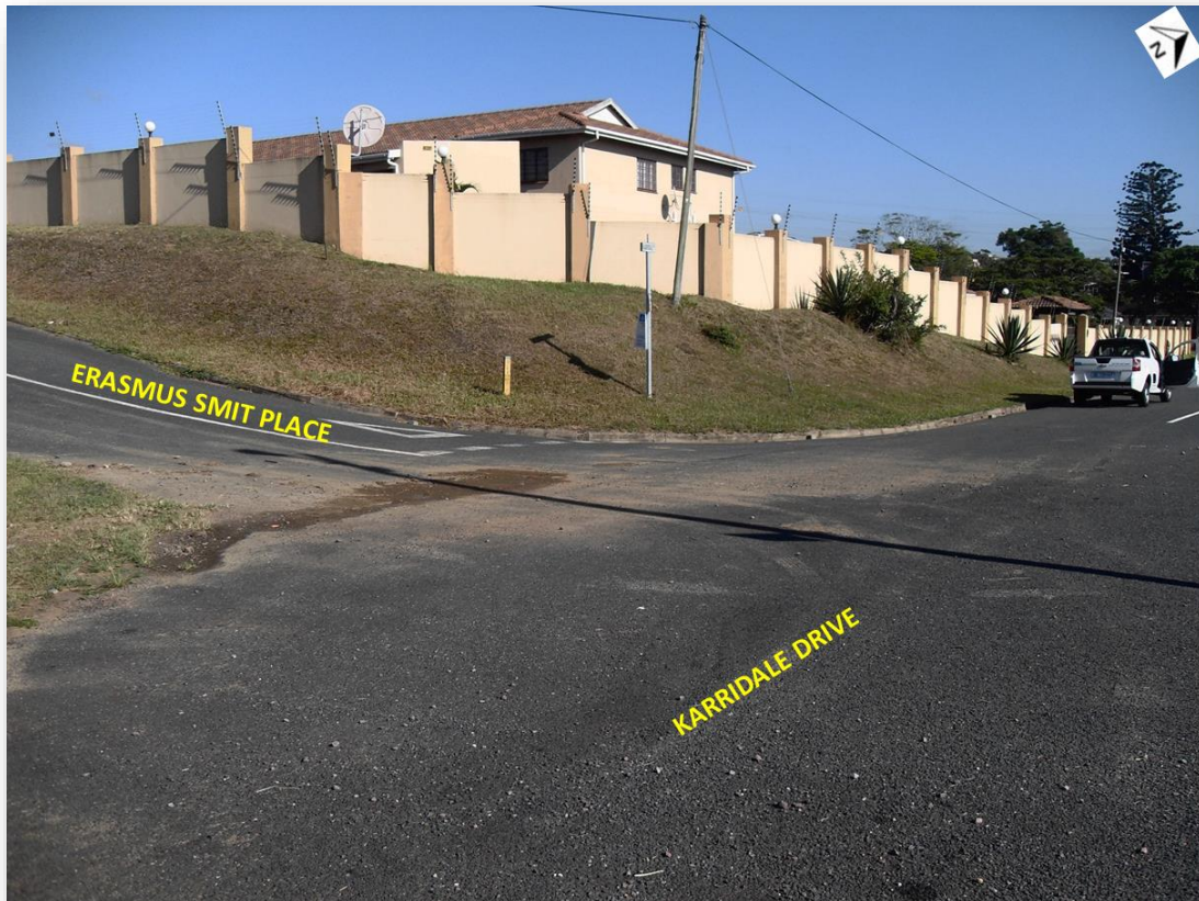
Figure 5: Intersection of Erasmus Smit Place and Karridale Drive facing north west
