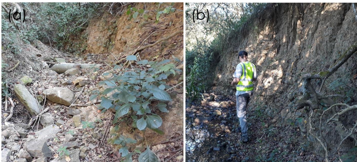
(a) Photograph showing of erosion along a storm water outfall that drains Longacre's Drive, which runs parallel to R01 with severe bank erosion and (b) Similar erosion features were noted at multiple locations along the course of stream R02.
